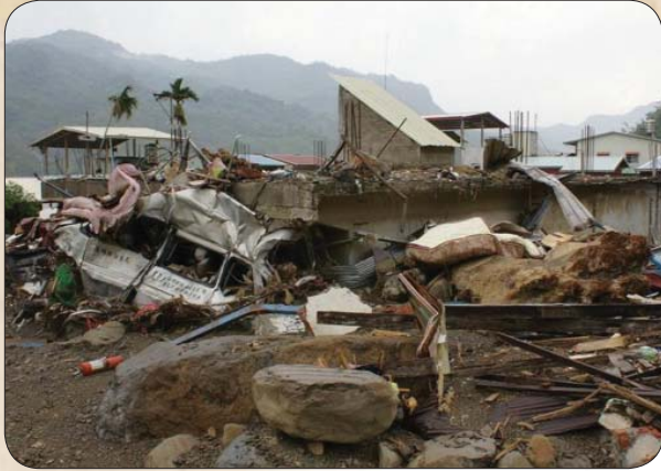
Typhoon Morakot caused extensive damage in many villages across southern Taiwan.
