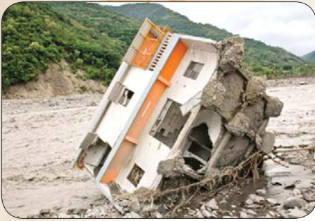
Homes and other buildings were torn from their foundations by raging waters fed by Typhoon Morakot.
